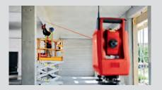
**Hilti Robotic Total Station:** Allows data flow from BIM to field and field to BIM. It enables guided single-person position layout and facilitates on the spot verification through linked material data with 3D fixing.
