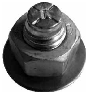
Figure 8 – Bolt head with length identification mark and KWIK Bolt TZ head notch embossment
