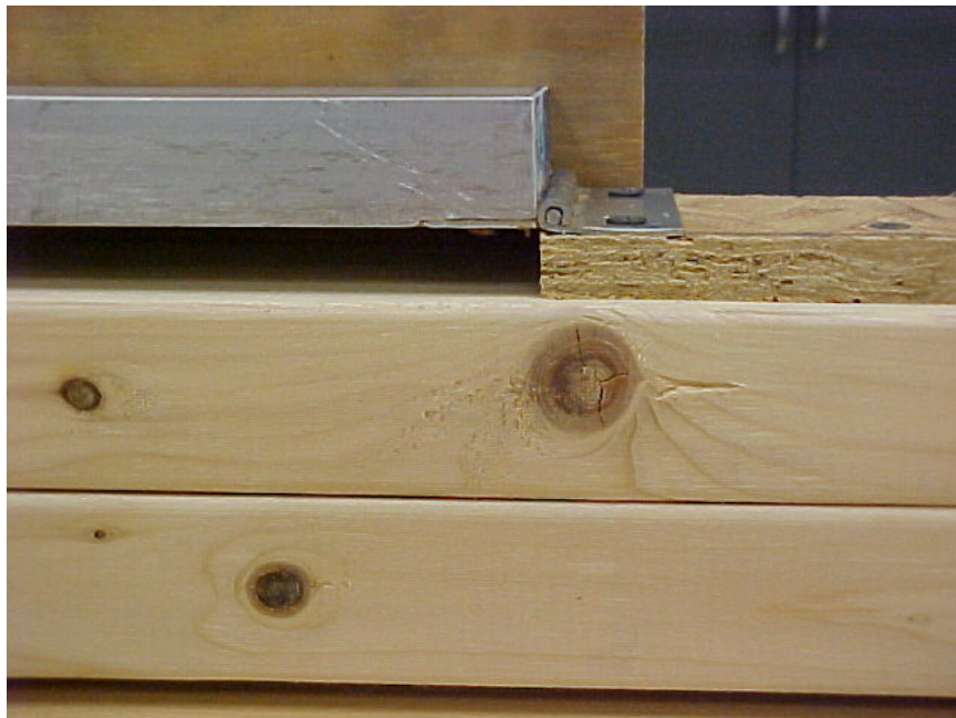
Photo No. 12 Beam Deflection Construct - Pinned Connection Detail
