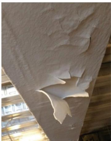
All repair MUST ensure that required DFT thicknesses are met as per UL requirements
