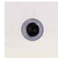
Pre-drill until the bit shoulder grinds a shiny ring (to ensure proper drilling depth).
