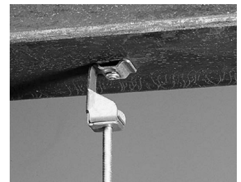
Threaded and smooth rod hangers
