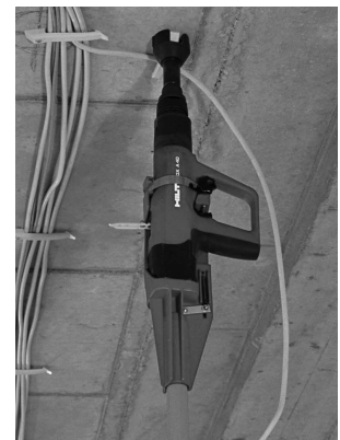
Cable and conduit attachment
