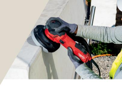
When used together with Hilti's new continuous rim, turbo-style diamond cup wheel, fast removal of overpour and a smooth finish are at your fingertips. Pair it with a compatible Hilti vacuum for an OSHA 1926.1153 Table 1 compliant dust control solution.
