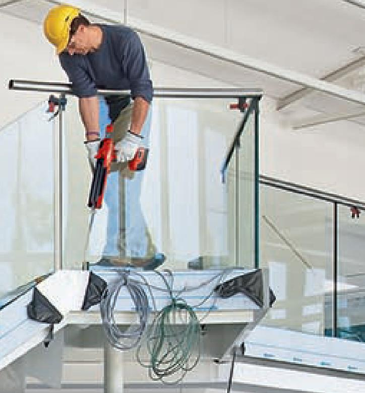
**The glass panes are supported with HIT-HY 270 from the base of the U-profile to the top of the U-profile in periodic locations along the length of the glass.**
