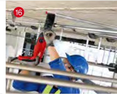
16 Post installed anchors
