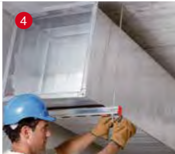
4 Mechanical & Electrical, HVAC
