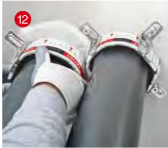
12 Piping and ventilation
