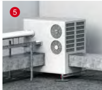
5 Air Handling Units
