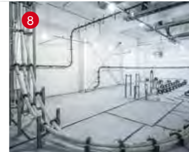
8 High voltage cabling supports
