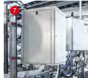
7 Equipment supports and platforms
