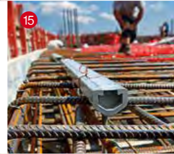
15 Cast-in anchors
