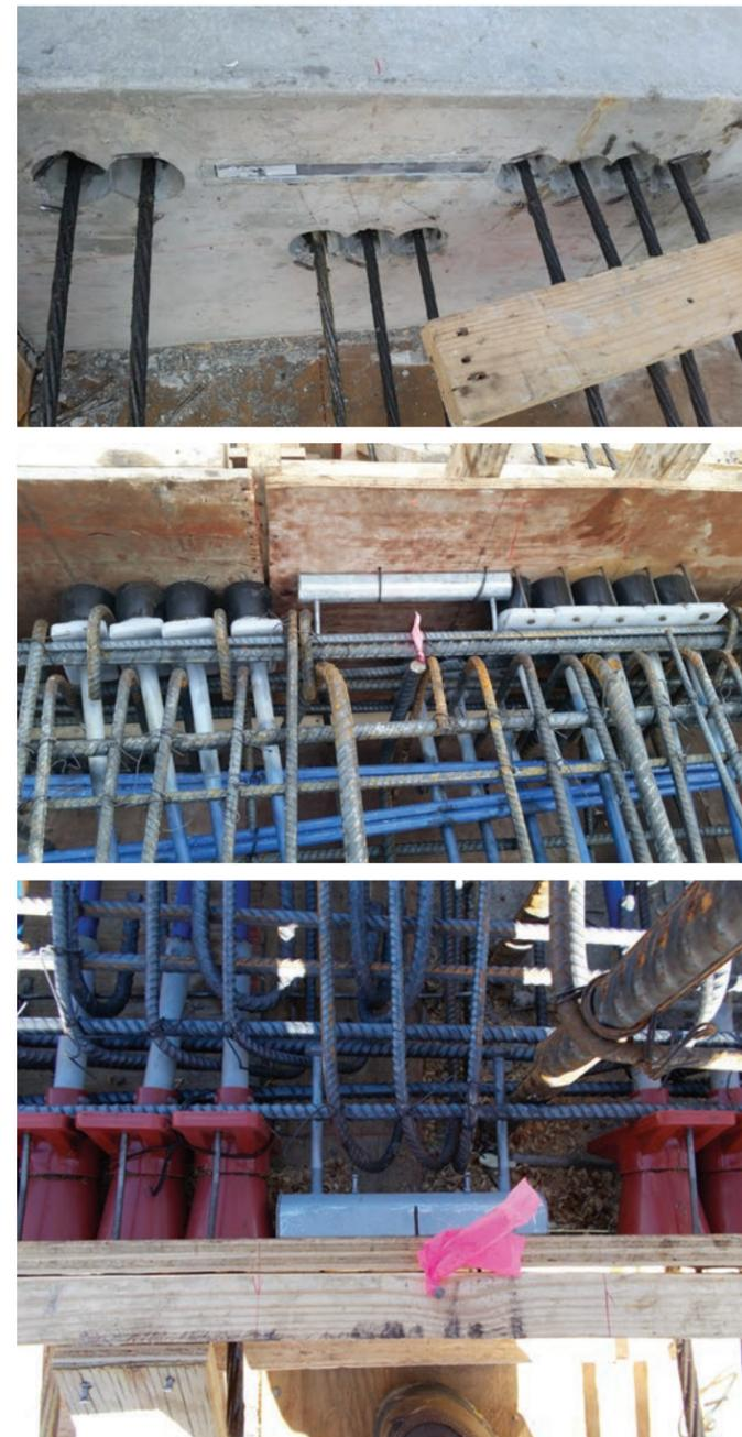
Figure 11.5.3.3 — Anchor channels installed near live end of post-tensioned cables. Contact Hilti for additional information.
