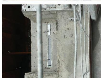
Figure 11.5.6.4 — Pictures of Conditions with Proper Concrete Consolidation at the Anchorage Zone.
