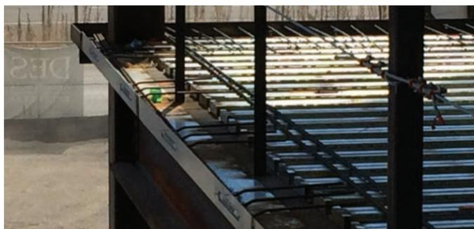
Anchor channel in composite slabs; face of slab application
