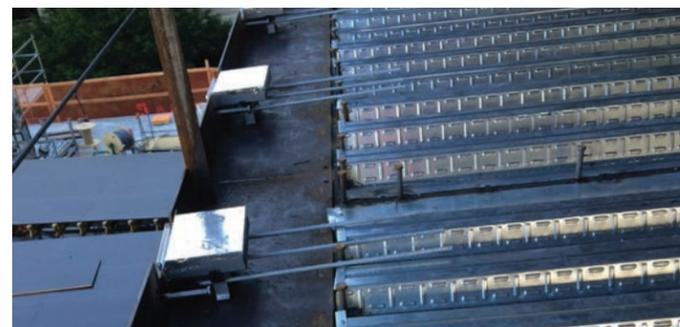
Anchor channel in composite slabs; top of slab application
