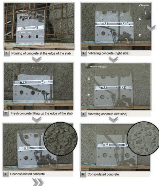
Figure 11.5.6.3 — Pouring and Vibrating Concrete at the Edge of the Slab.
