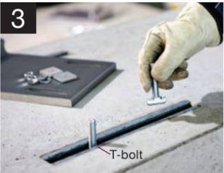
T-bolts can be installed along the channel length (except outers 1"), thus allowing for the so desired installation tolerance.
