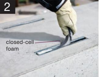
The closed-cell foam allows for an easy tear out strip, allowing the entire foam length to be continuously removed.
