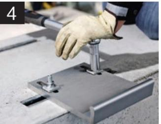
Fixture is positioned in the proper position and the hexagonal nut is tightened to the right setting torque.
