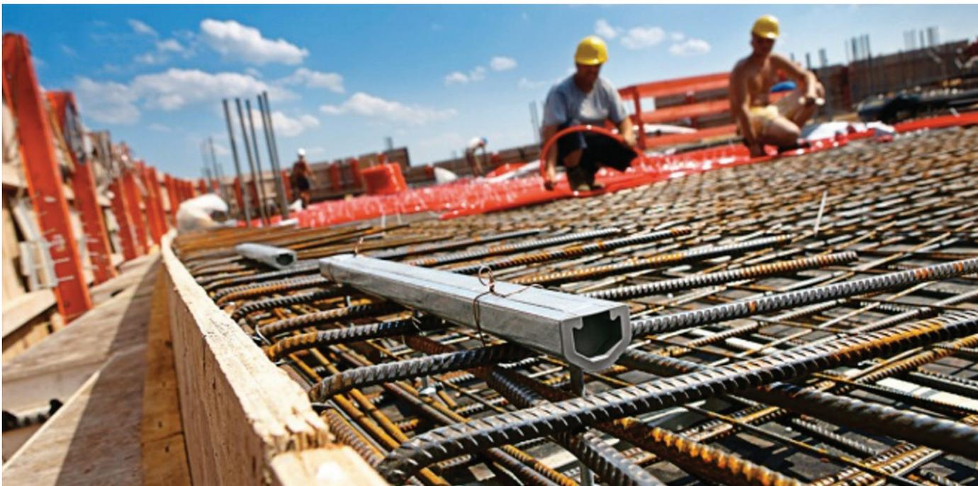
Anchor channel in the slab prior to casting of the concrete.
