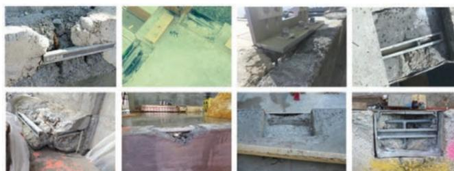
Figure 11.5.6.1 — Pictures of Conditions with Improper Concrete Consolidation at the Anchorage Zone.
