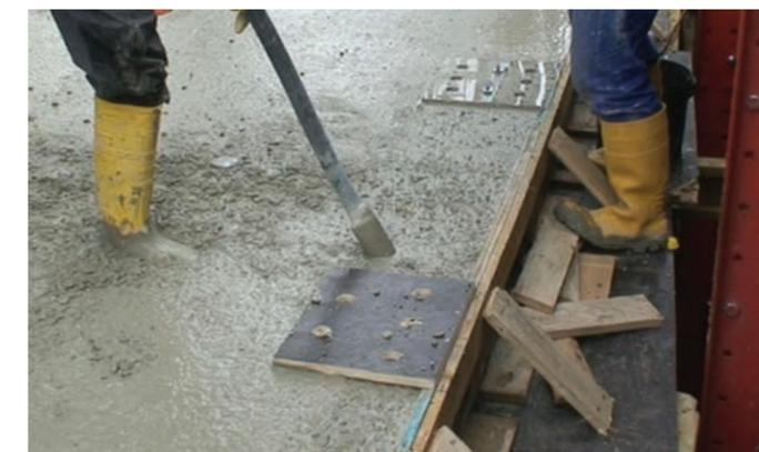
Figure 11.5.6.5 — Construction Member Vibrating the Concrete at the Anchorage Zone.
