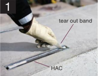
The tear out band simplifies the foam removal.
