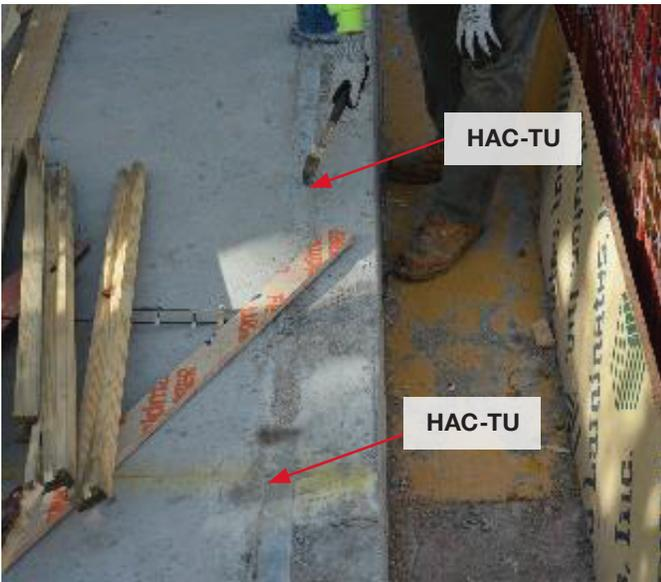
Figure 2 — HAC-TU cast-in concrete
