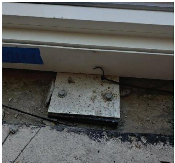
Figure 8 — Window Wall façade frame fastened via HAC-TU and Self-drilling screws
