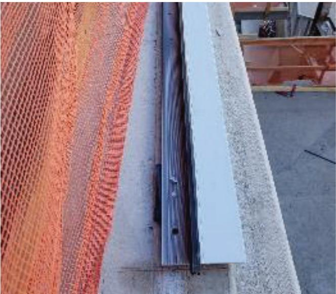
Figure 3 — Window wall sill connected via HAC-TU
